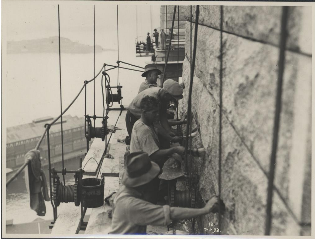
Workers on the south-western pylon of the Sydney Harbour Bridge. Sidney. 1922-1932. Museum of Applied Arts & Sciences . Via Flickr. Document sense restriccions conegudes de drets d'autor.
