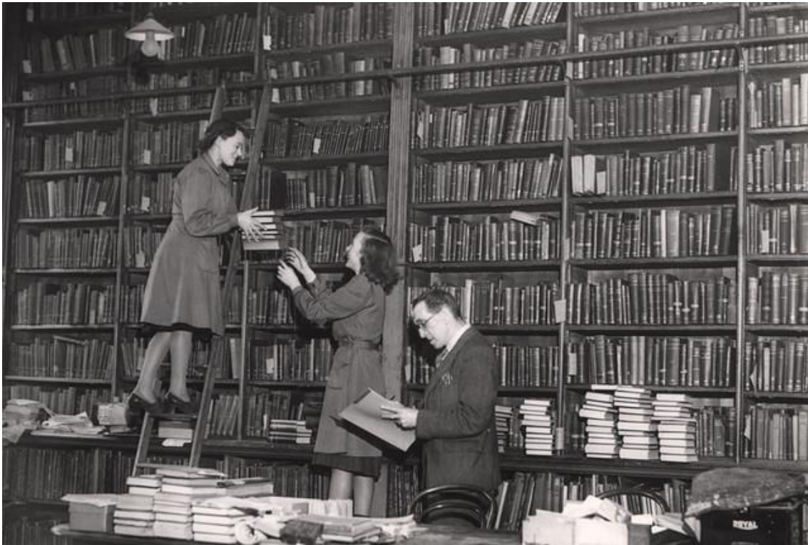
Temporary Lending Library Central Library New Bridge Street Newcastle upon Tyne. 1949. Newcastle Libraries . Document en el domini públic.
