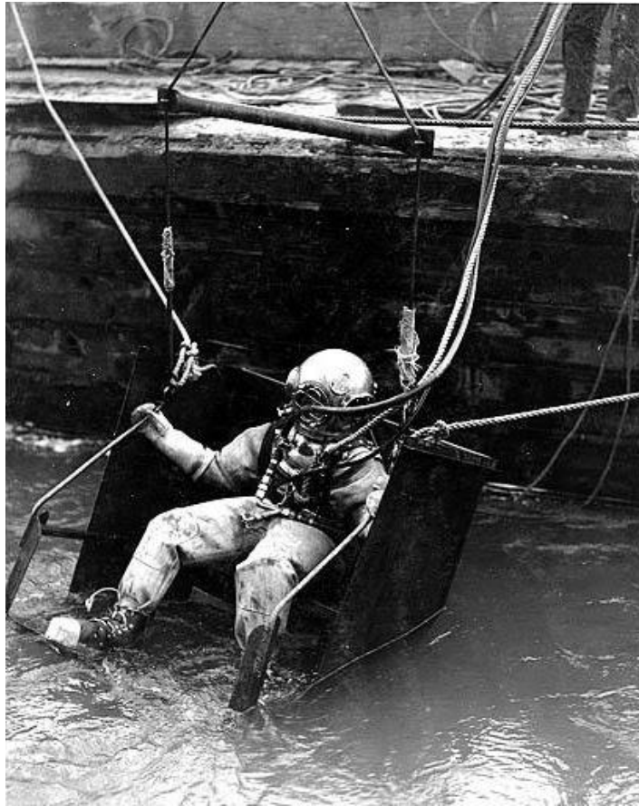
Diver entering water, Grand Coulee Dam construction site. Estats Units (Washington). 07/01/1938. University of Washington Libraries . Document sense restriccions conegudes de drets d'autor.
