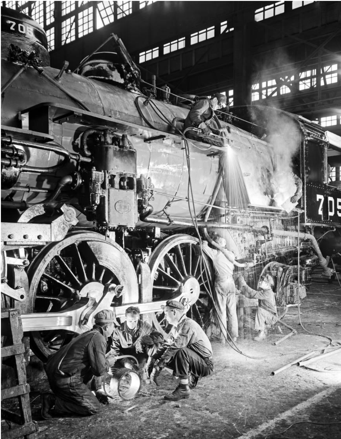
Robert Yarnall Richie. Work Crew Repairing Locomotive 705, Texas & Pacific Railway Company. 1946. SMU Central University Libraries . Document sense restriccions conegudes de drets d'autor.
