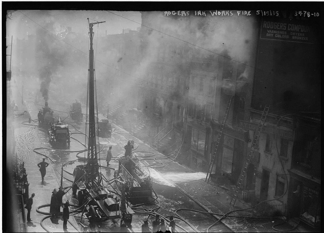
George Grantham Bain. Rogers Ink Works fire . 1915. The Library of Congress . Document sense restriccions conegudes de drets d'autor..
