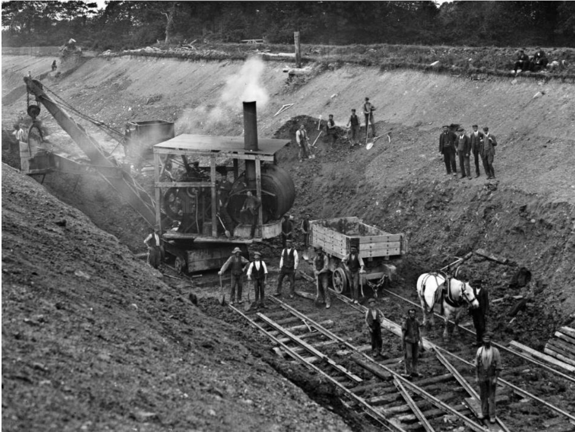
A. H. Poole. Mr. Cuthbert, New railway, Gracediew, cutting. 1905. National Library of Ireland . Document sense restriccions conegudes de drets d'autor.
