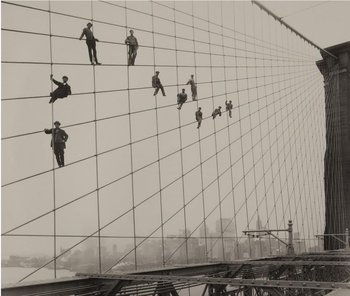
Eugene de Salignac. Painters on the Brooklyn Bridge Suspender Cables-October 7, 1914 . 1914. Museum of Photographic Arts , via Flickr . Document sense restriccions conegudes de drets d'autor.
